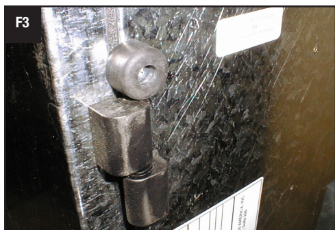
Rubber Door Keeper installed on Blower Access (large) Door.
