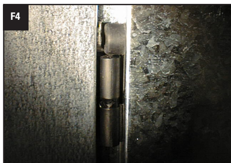
Rubber Door Keeper installed on Filter Access (small) Door.
